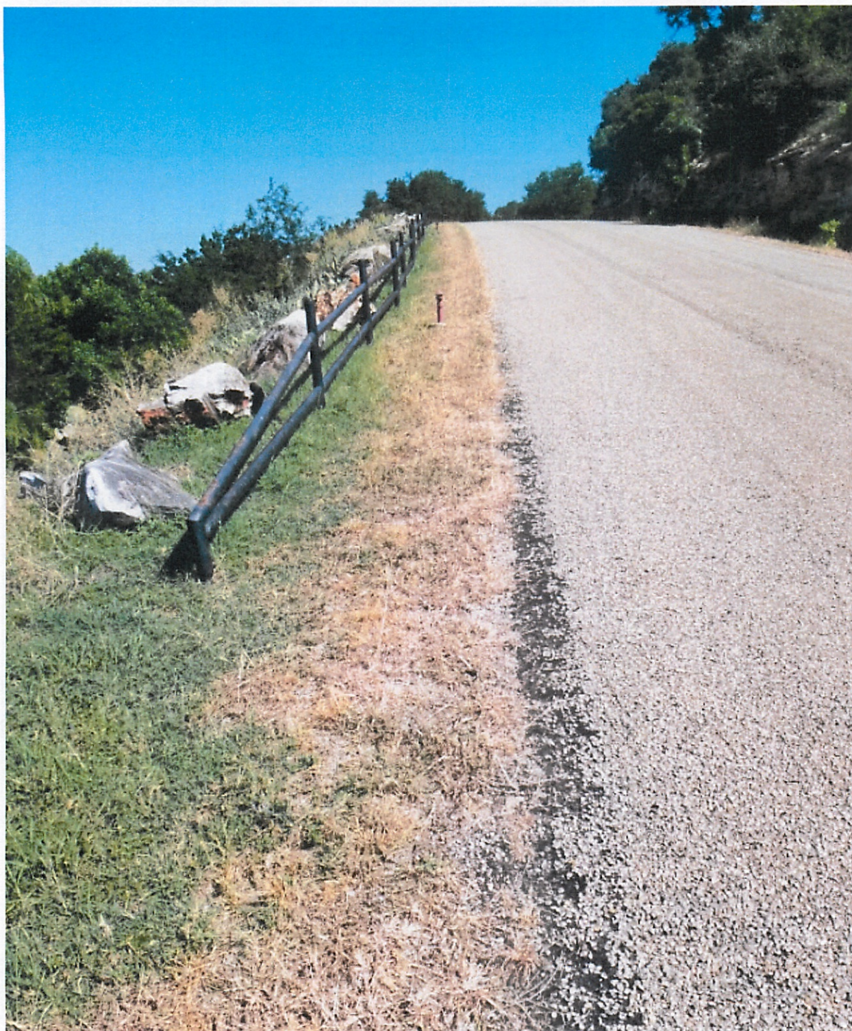
Unauthorized spraying on Wolf Creek Ranch Road (adj to MCW-2)
