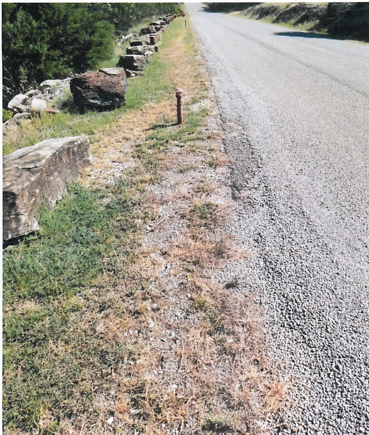
Unauthorized spraying on Wolf Creek Ranch Road (adj to MCW-2)
